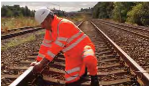
Using a track-circuit operating clip
