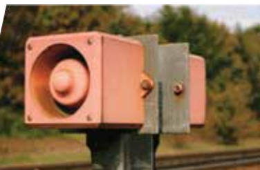
Example of a TOWS warning siren
