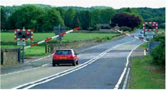
Automatic half-barrier level crossing
