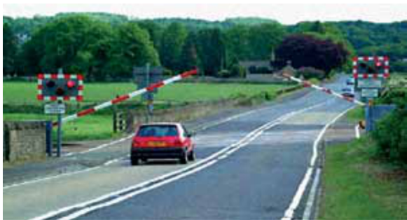
Automatic half-barrier level crossing
