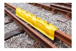
NOTE: the number of conductor rail shields used would normally be limited to the number which may safely be removed before the passage of a train; normally this number would not exceed more than one shield for each member of staff on site, excluding lookouts and site wardens.
