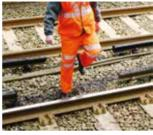
Cross at a conductor rail gap wherever possible
