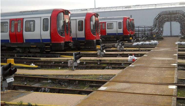
Using walk boards is the safest method of crossing the track in depots and sidings. Walk boards:
