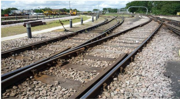
These are sections of track which do not have conductor rails, normally found at the ends of the lines or within certain depots and sidings. Due to the nature of these lines having no traction current rails, Engineering Hours does not apply. At these locations, Traffic Hours/depot protection or a possession is required to access the track.
